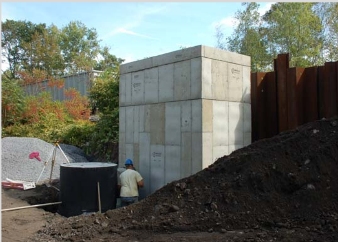
Precast Overflow Chamber in position, Moosic, PA
