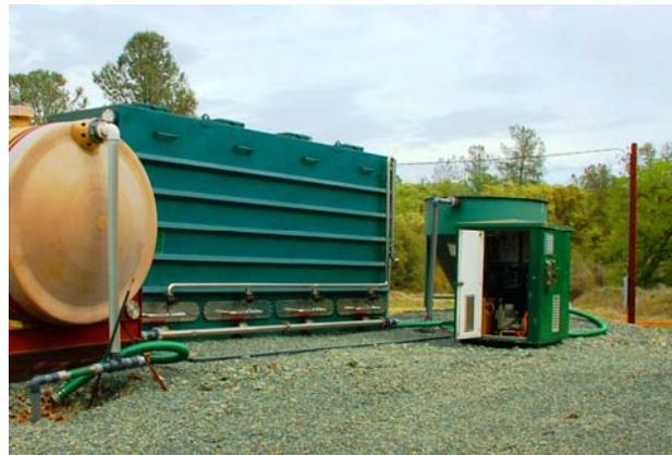
SAF at Yuba Co. with Septic tank in foreground and control kiosk and secondary clarifier in background.
