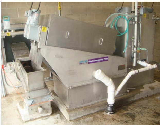
The Volute Dewatering Press is designed to be fully automated, capable of starting up, operating, and shutting down with no operator intervention.
